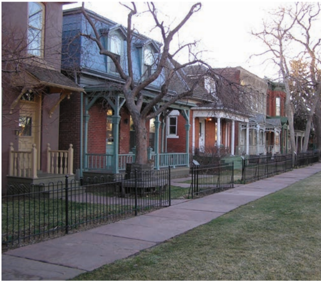
AHEC has received a large grant from the Colorado Historical Society at History Colorado. The grant will fund Historic Structure Assessments on the thirteen buildings located in the Auraria 9th Street Historic District so they can continue to honor the past into the future.
