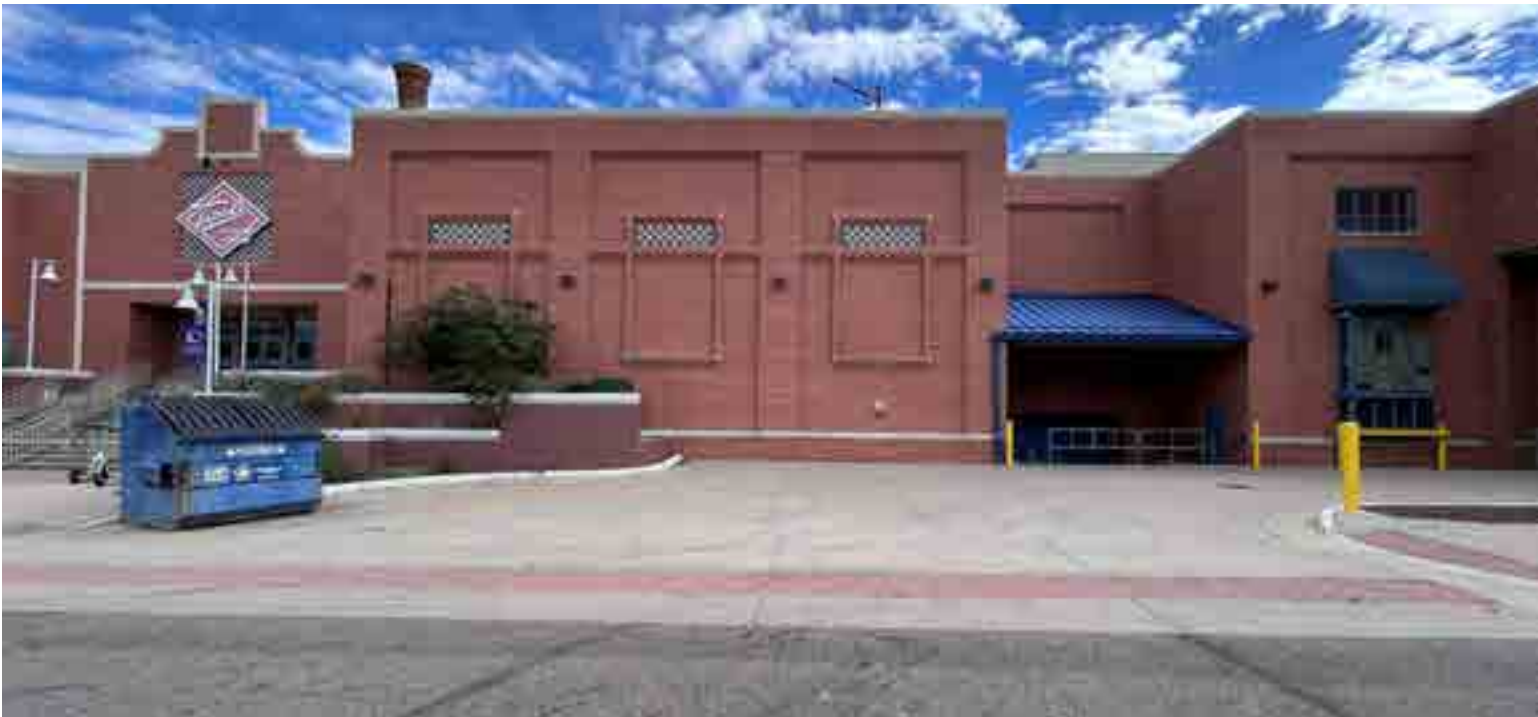
The Tivoli's West Facade Includes a Main Entry (left), waste pickup (center), and freight deliveries (right)
